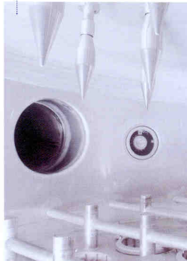
Niro SANICIP™ Bag Filter. Clean air plenum.
