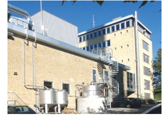
Solvent vapour adsorption and waste water tanks
