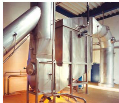
Process thermal heat recuperator unit and ducting equipped with CIP nozzles
