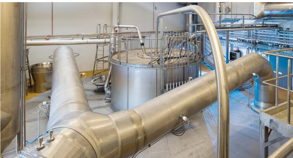
Process thermal heat recuperator unit and ducting equipped with CIP nozzles
