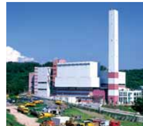
A Taiwanese waste incineration facility with two Niro SDA systems, 2 x 300 TPD.
