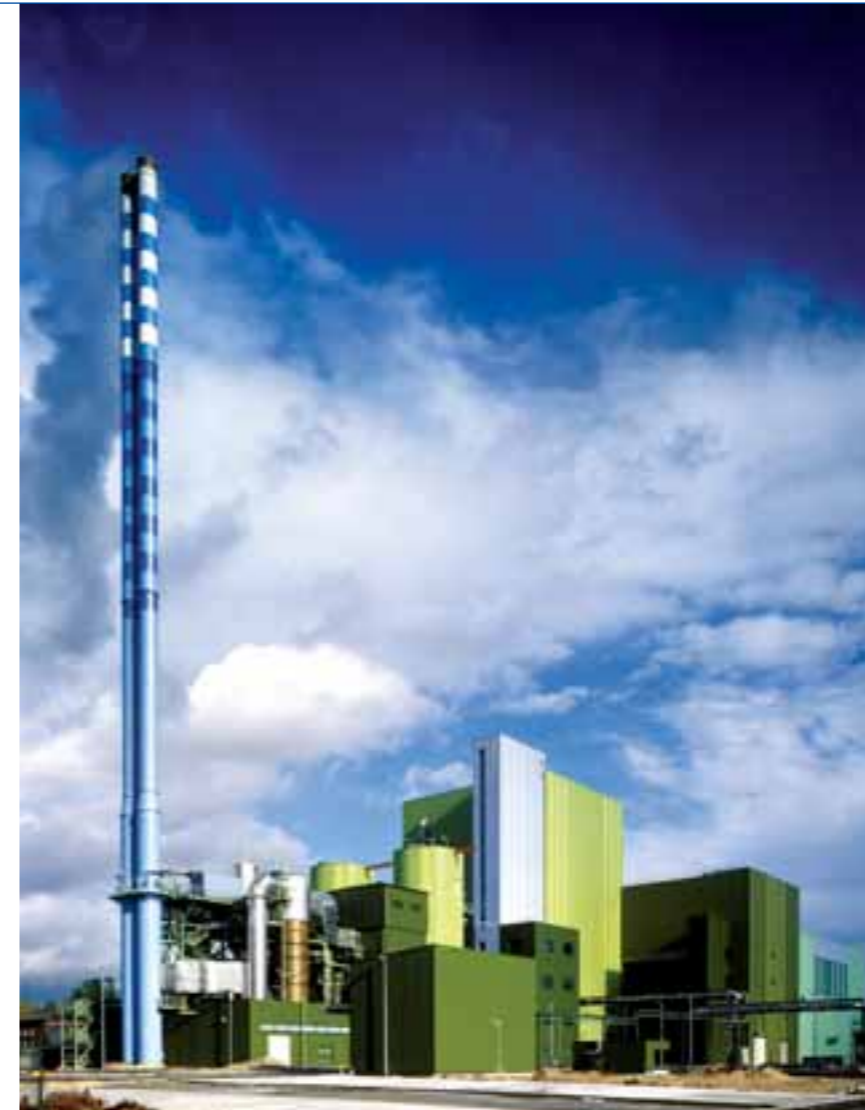
A Niro SDA system in combination with polishing wet scrubbers at two waste incineration lines in Germany, 2 x 300 TPD.
