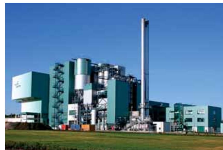
Two waste incineration lines in Germany, 2 x 300 TPD.
