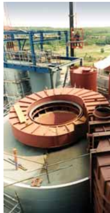
Erection of a gas disperser at a German incineration plant.
